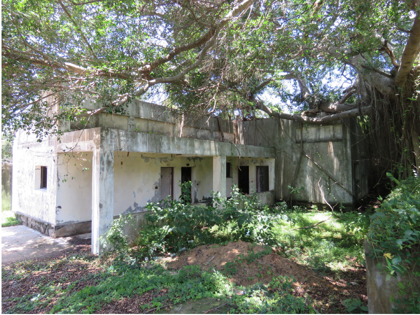
Figure 2.1. A disused building of a former military brothel in Anqian, Kinmen, 2018. © Hsiao-Chiao Chiu.
