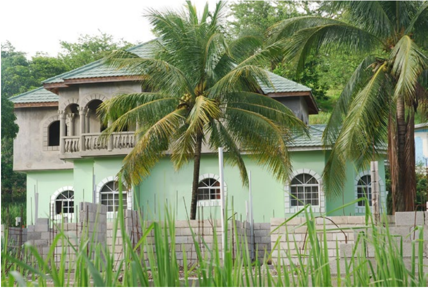
Figure 13.1 Hillside house with columns. In this example, the top floor has recently been added to an existing single-storey house, and the fashion for elaborate columns has been included in the later part of the design. Photograph by Davinia Gregory, July 2013.
