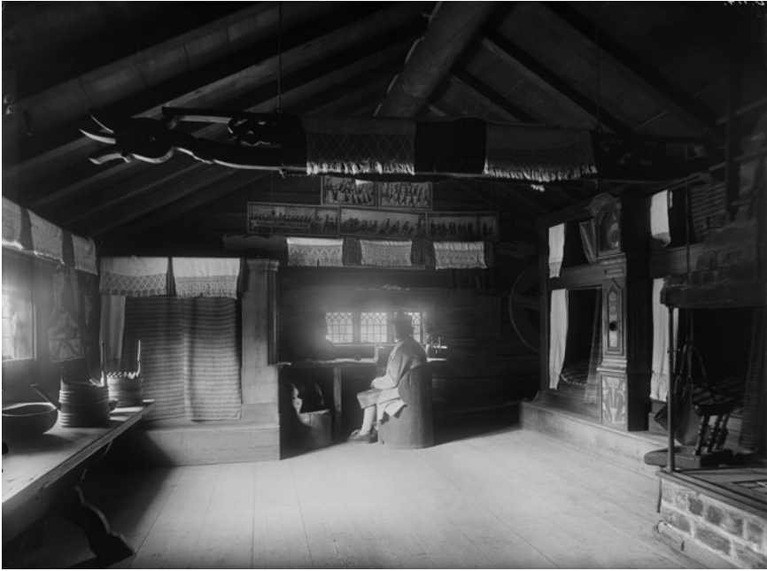
Fig. 10.2 Interior view of the eighteenth-century Morastugan – the first building to be relocated to Skansen, forming a key part of the museum from its opening in 1891. Photographer unknown. Courtesy of Stockholm Stadsmuseum.
