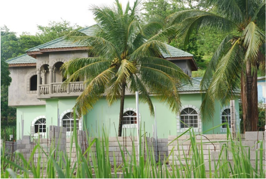
Figure 13.1 Hillside house with columns. In this example, the top floor has recently been added to an existing single-storey house, and the fashion for elaborate columns has been included in the later part of the design. Photograph by Davinia Gregory, July 2013.
