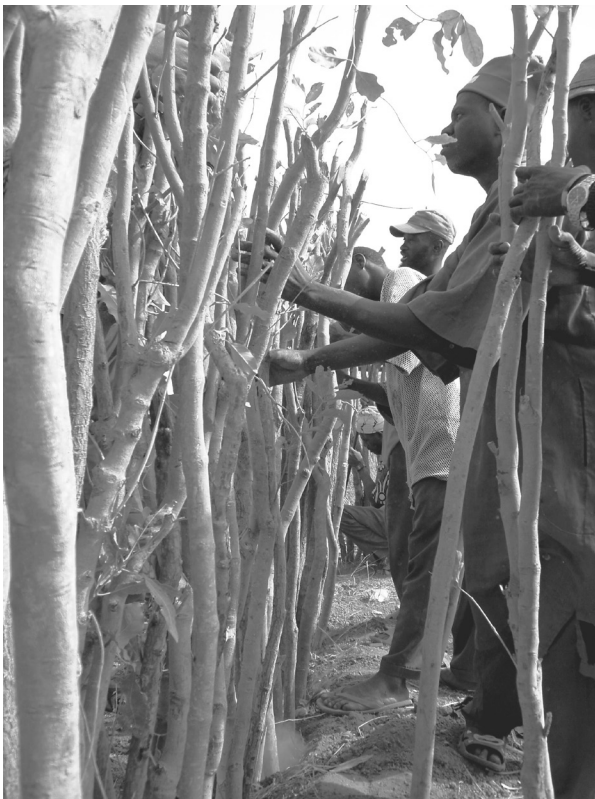
Figure 6.1 Building Civic Responsibility: Restoring the Fence of a Stable for Horses and Donkeys Caught Wandering in the Village at Night, 2008
