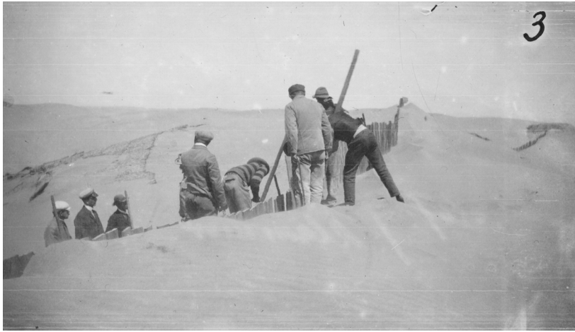
Figure 6.4. NAN 28723, “Construction of the railway line Lüderitzbucht-Keetmanshoop. Dune protection wall: Lifting the wall planks, 1909,” courtesy of the National Archives Windhoek.
