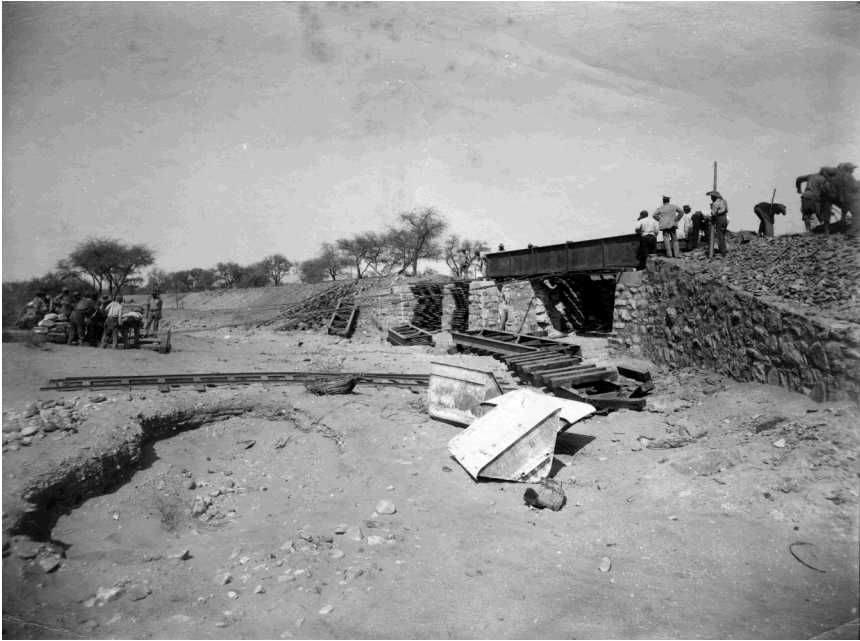
Figure 3.4. NAN 23383, “Railway bridge construction, probably between Windhoek and Swakopmund [190?],” courtesy of the National Archives Windhoek.
