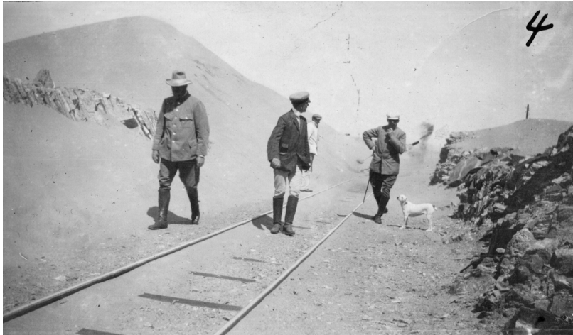
Figure 6.5. NAN 28724, “Construction of the railway line Lüderitzbucht-Keetmanshoop. Inspection of railway tracks threatened by sand dunes, 1909,” courtesy of the National Archives Windhoek.
