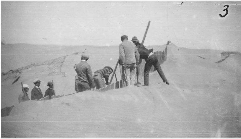
Figure 6.4. NAN 28723, “Construction of the railway line Lüderitzbucht-Keetmanshoop. Dune protection wall: Lifting the wall planks, 1909,” courtesy of the National Archives Windhoek.
