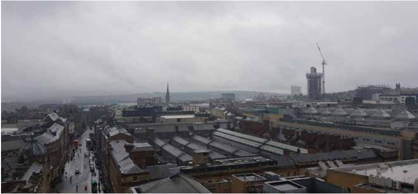
Figure 8.1. Hadrian's Tower under construction, in Newcastle upon Tyne. © Sarah Winkler-Reid
