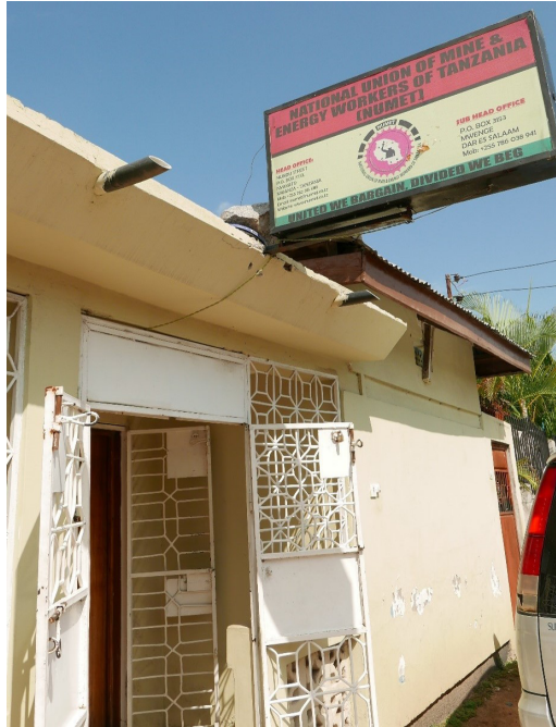
Figure 8.2. The office of the National Union of Mine and Energy Workers in Tanzania (NUMET). The staff at Equinor Tanzania established a union branch under NUMET. The branch leadership were taken to Norway for “capacity building.” © Siri Lange.
