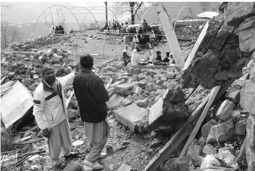
Figure 1.1. A Collapsed School. A community member indicates how, in the earthquake, the Government Girls' High School Kheral Abbasian collapsed. Students continued attending class in the rubble. 2010. © Jane Murphy Thomas.
