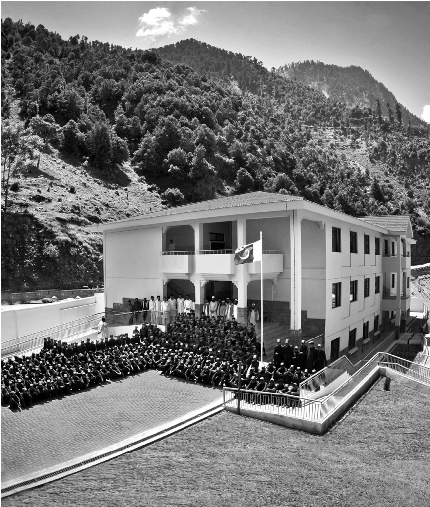
Figure 1.2. Mohandri School. At this location, the earthquake dislodged boulders, which rolled down the nearby steep mountain slope, smashing into the school, taking several lives. Here, students and teachers pose in front of their new school constructed by the PERRP project. Government Boys' Primary and Secondary Schools, Mohandri village, Khaghan Valley, KP. See anecdote in Chapter 6: "Mohandri School, Mountainside Boulders." 2011. © Umar Farooq.
